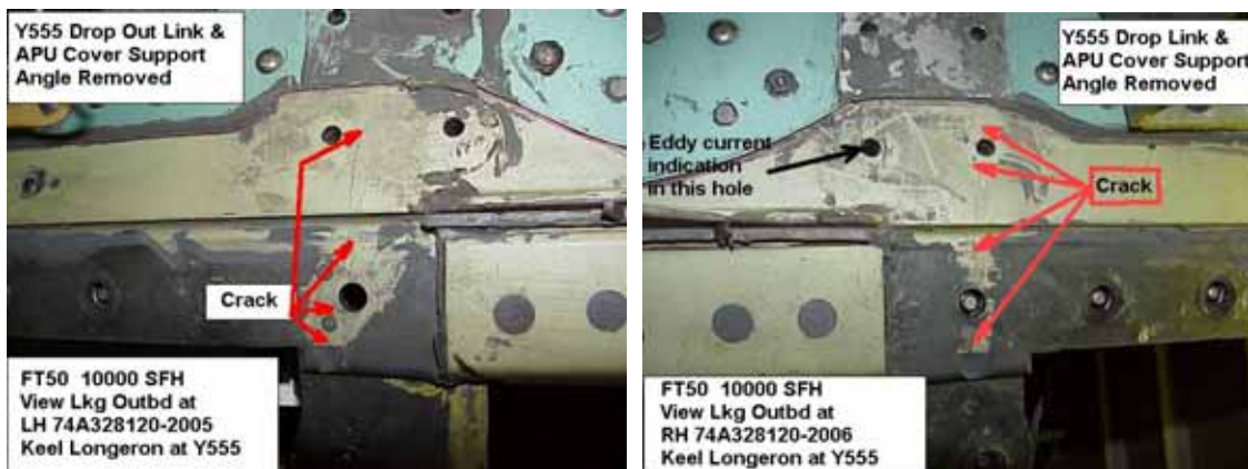
Figure 9 – Keel longeron Y555 cracks at 10,000 SFH
