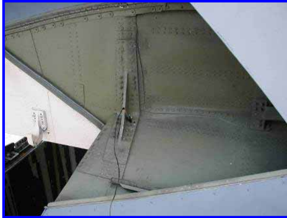
C-5 Contour Box Beam Fitting (CBBF) Structure
